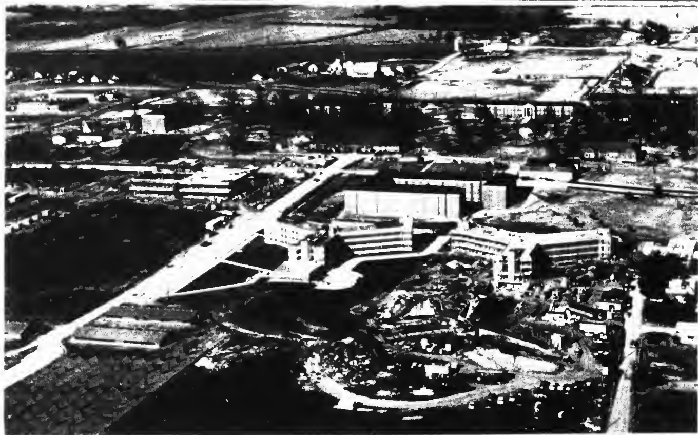
An aerial photograph of the campus gives a complete view of construction now in progress and shows the site of the library soon to be built, indicated by the patch.
